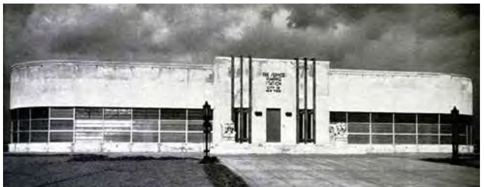
The masonry above the windows is suspended by cantilevered ends of the Pumping Station's roof girders. (Source: Short and Brown, 1939, Public Buildings)
