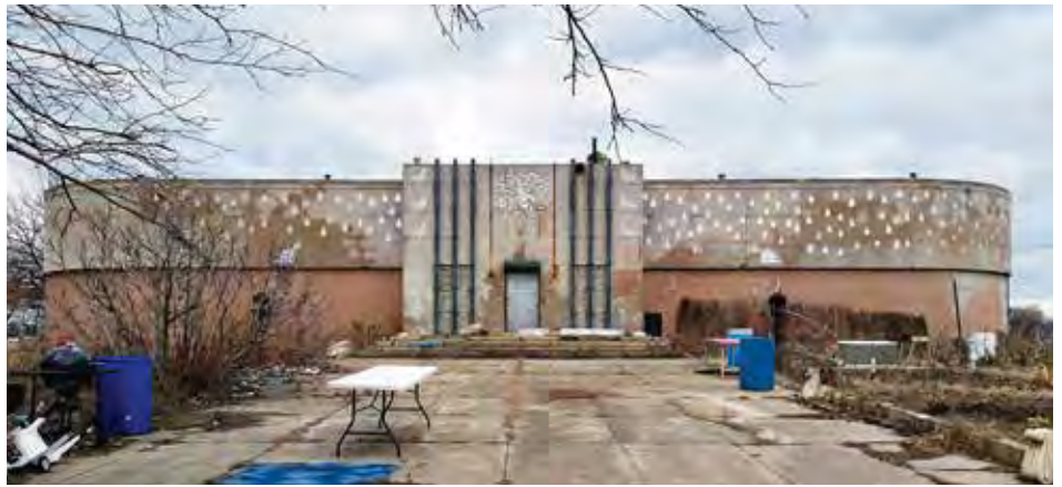
Despite years of neglect, the wide walk between lawns leading to the entrance of the curvilinear Coney Island Pumping Station still conveys Irwin S. Chanin's stately Art Moderne design. When the continuous band of three-tier windows (see below) was damaged by vandalism, the City installed painted cinder blocks to protect the building. (Courtesy of Flickr/Matt Green)
